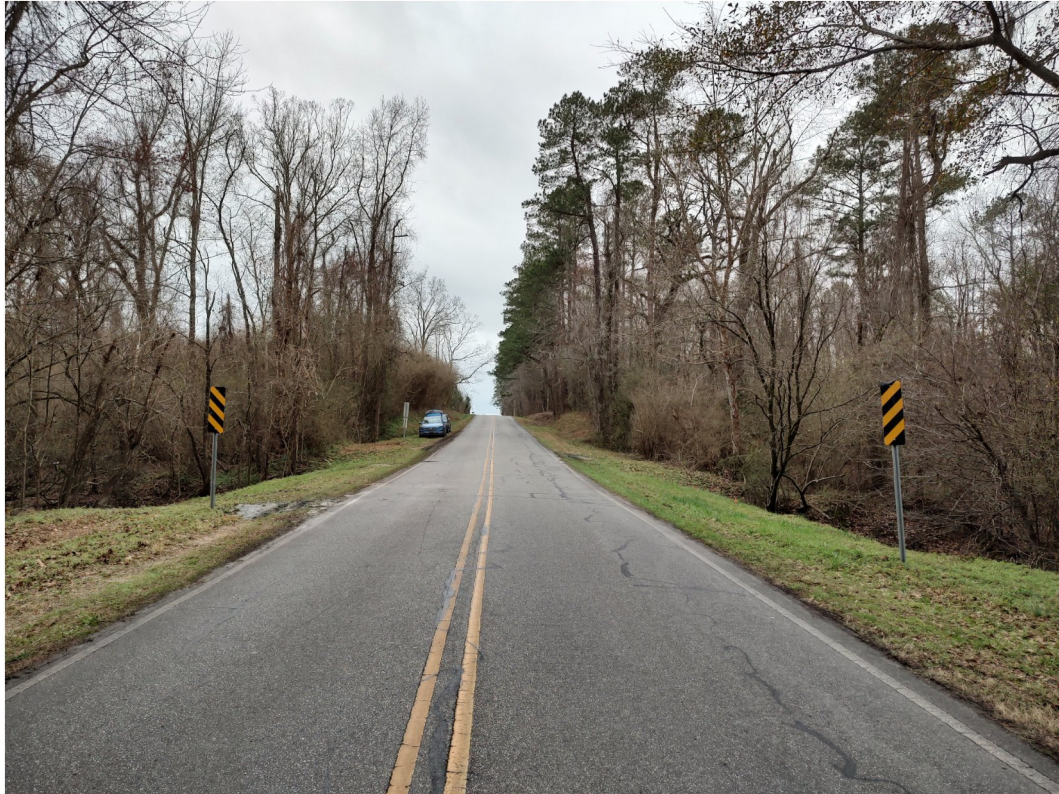
PHOTO 1 - VIEW DOWNSTATION FROM END BENT 2.
