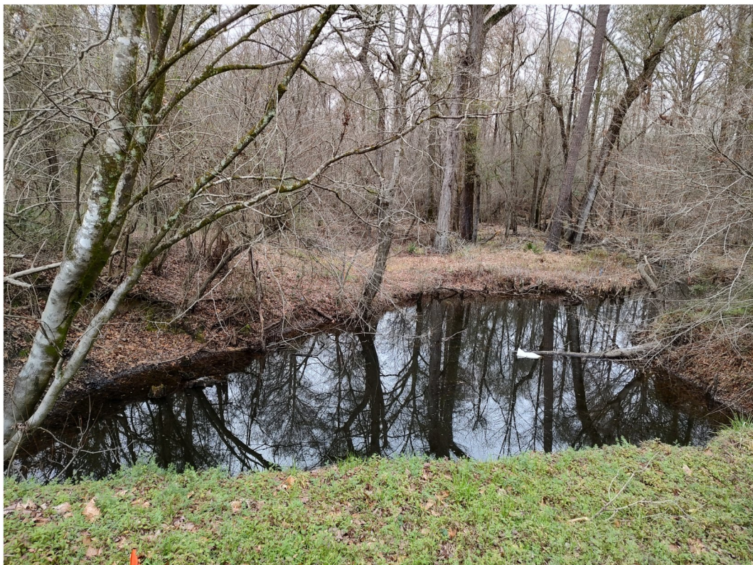
PHOTO 2 - VIEW FACING DOWNSTREAM FROM THE STRUCTURE.
